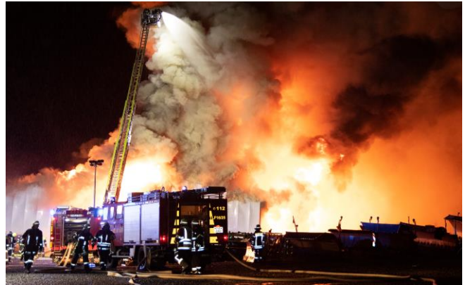
Brand Kasonhalle Eisensteg
